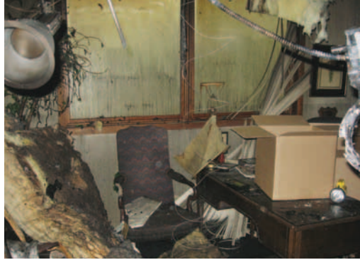
Physician's office prior to renovations.
